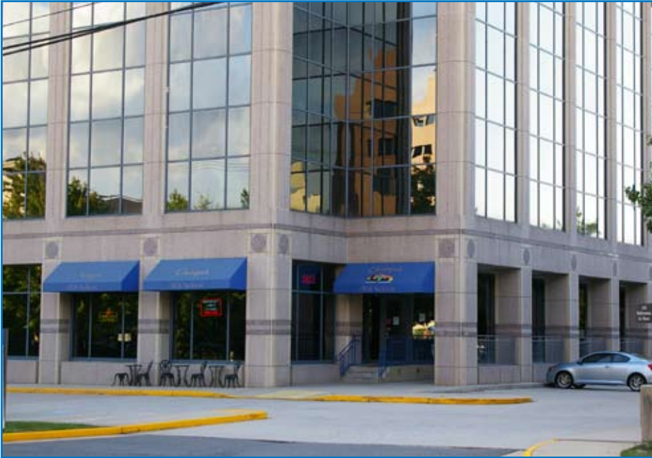
8100 Boone Boulevard - International Gateway I
