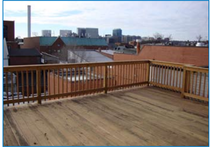
Roof Top Deck
