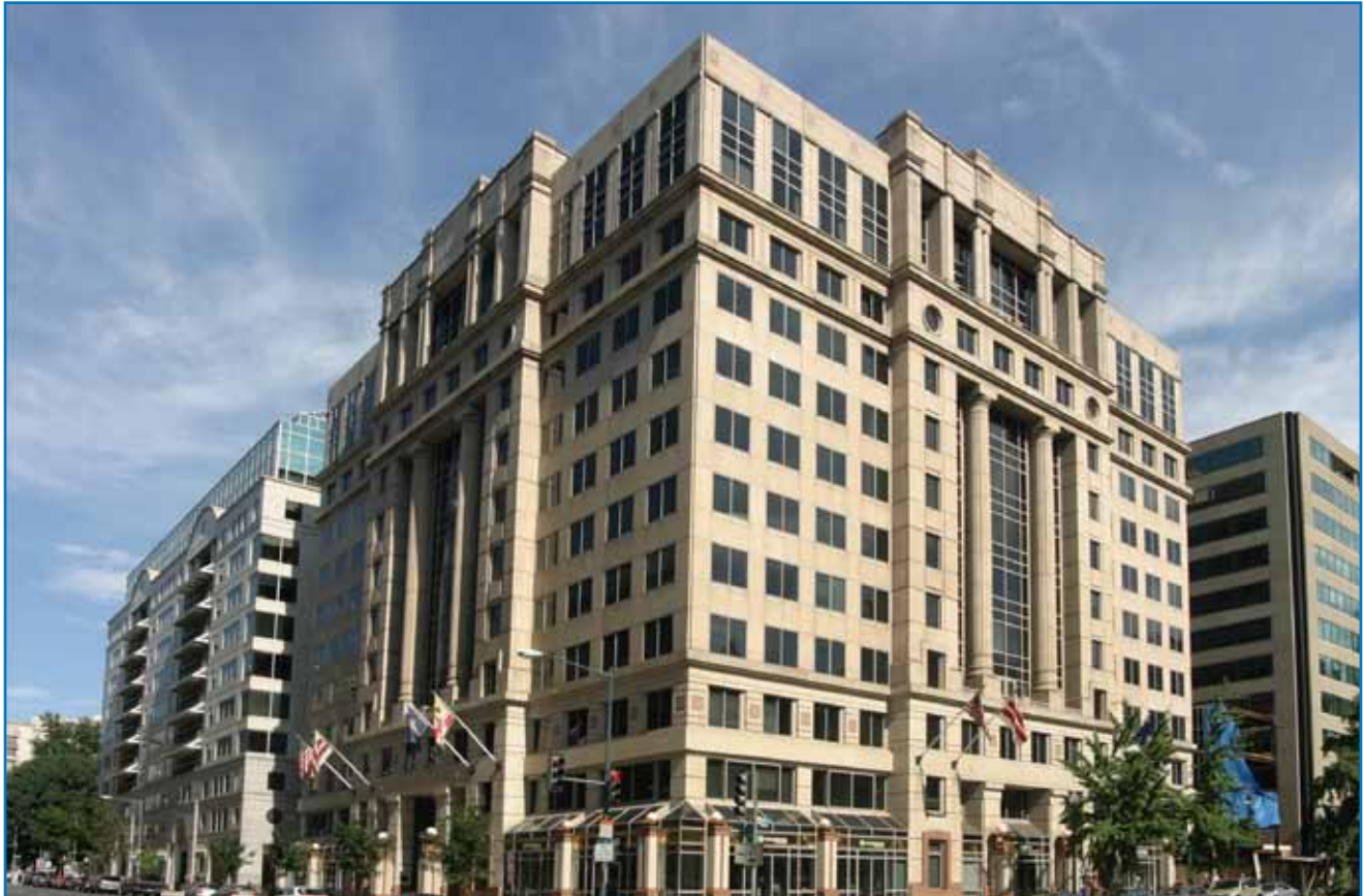
Franklin Tower—1401 Eye Street, NW
